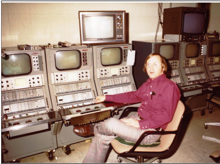
FIGURE 6. Color camera setup and shading operations in the 1970s. (These camera control units (CCUs) were used with Norelco PC-70S cameras.)
