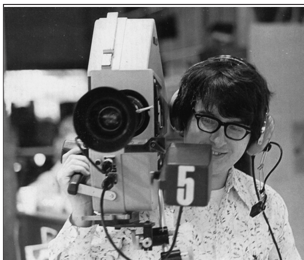
FIGURE 2. RCA’s TKP-45 “minicam” was released in 1975 and saw much during the 1970s and beyond. With lens and viewfinder, it weighed 25 lb and required an external power source.
